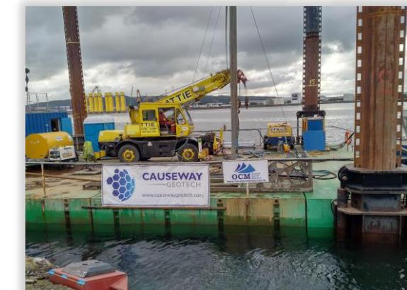
Rotary drilling works underway at a marine borehole location
