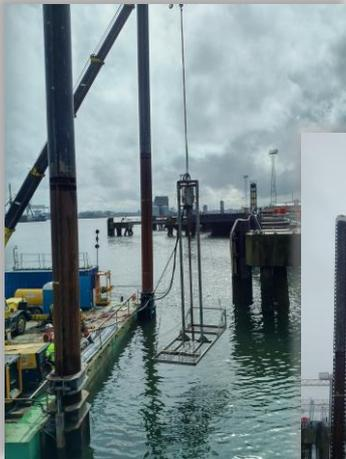
A vibracore sampler being lowered into the water at location within VT2 berth
