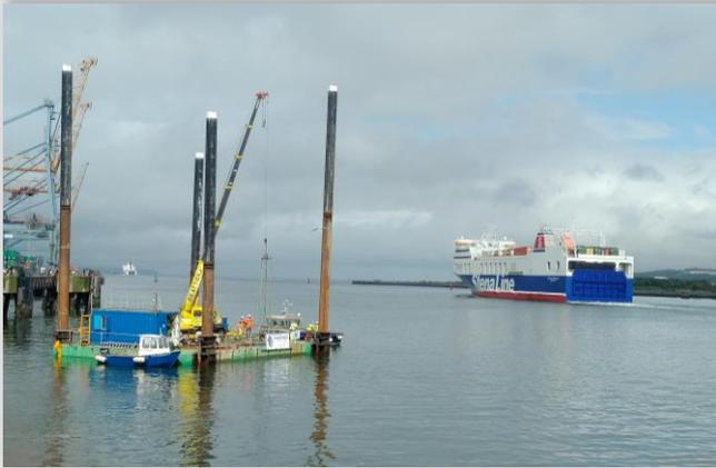
Jack-up barge set-up in position over a borehole location within Belfast Harbour
