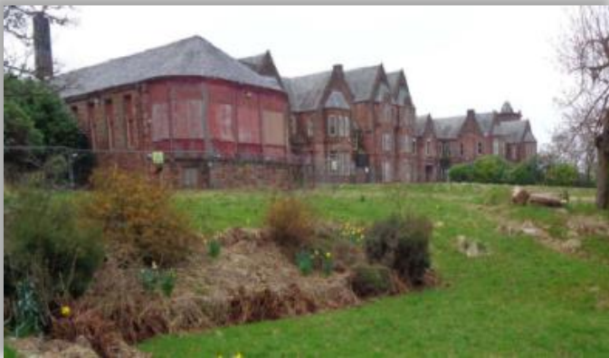
The derelict Smithston Building located in the south-west of the site (Fairhurst, 2016)
