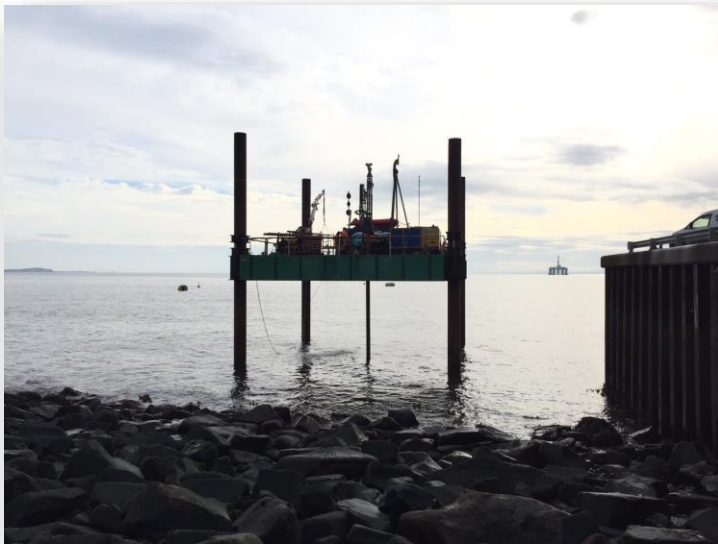
Drilling works underway at a nearshore borehole location
