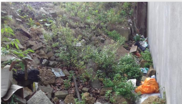
Access restrictions to hand pit locations along an existing retaining wall
