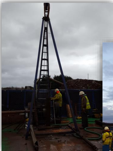
Jack-up barge set-up in position over borehole location
