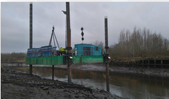
Drilling works underway at a riverbank borehole location
