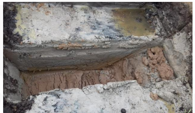
Trial pit excavations: wide, shallow excavation to allow access for detailed logging in upper strata.
